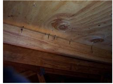
Marks showing locations of fasteners
