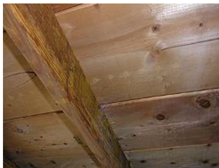
Planking roof deck (click image for larger version)
