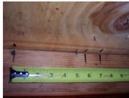
Measure the largest distance between fasteners
