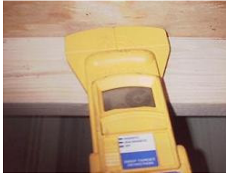
Using metal detecting stud finder to locate fasteners in rafters or truss top chords
